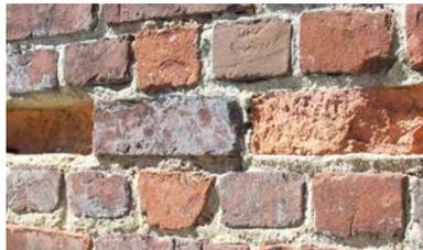
*a spalled brick face exposes the clay body to the elements and may cause substantial damage if left unrepaired.*
