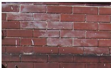
*efflorescence requires soluble salts and a water source. The likelihood of efflorescence varies according to the composition of the clay used to form the bricks.*
